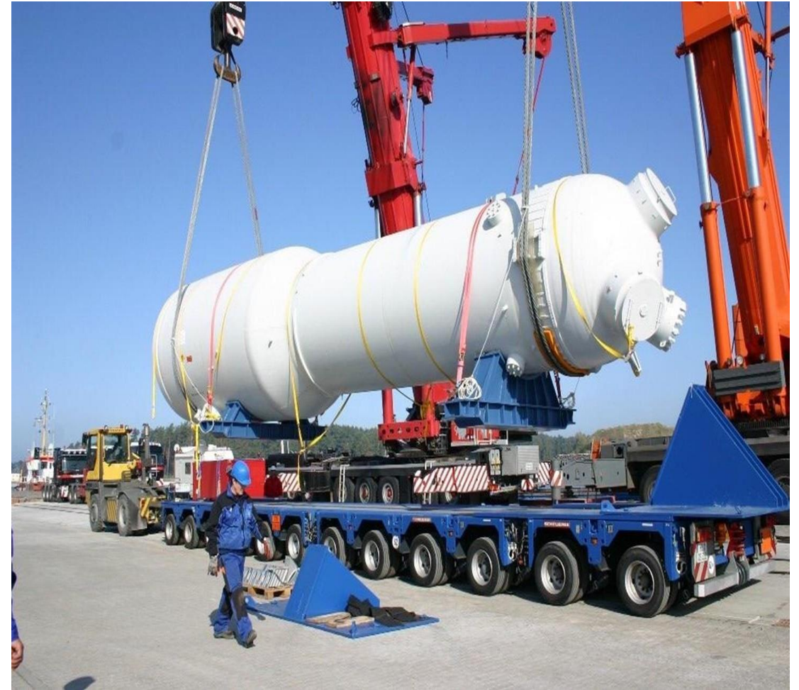
Original Steam Generator
